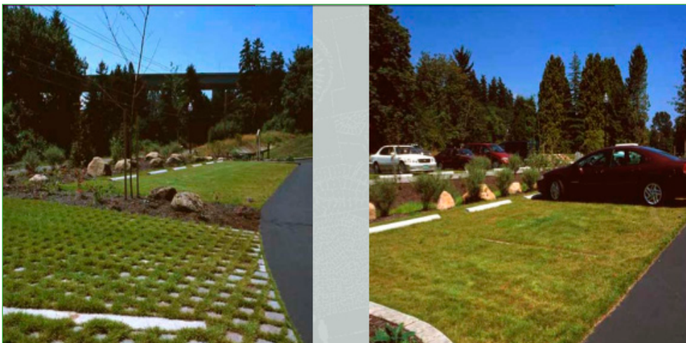
Turf Block and Paver Mat (Alameda CCWP, 2006)
